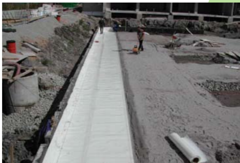
Compacted Sand Blinding
