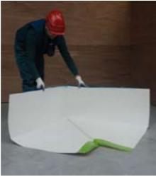
Fold internal corner & tape
