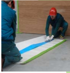
Measure, crease & fold membrane
