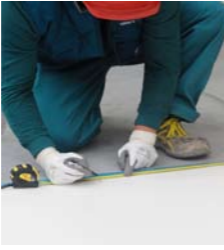
Measure, crease & fold membrane
